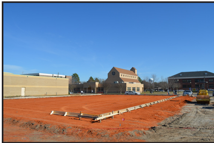
Groundbreaking/Construction site of the new Student Health & Wellness Center
